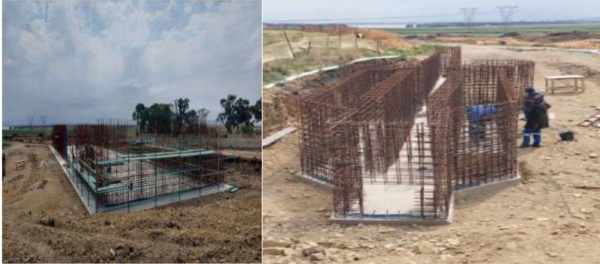
Upgrading of Orangeville Wastewater Treatment Works WWTW (WSIG)
