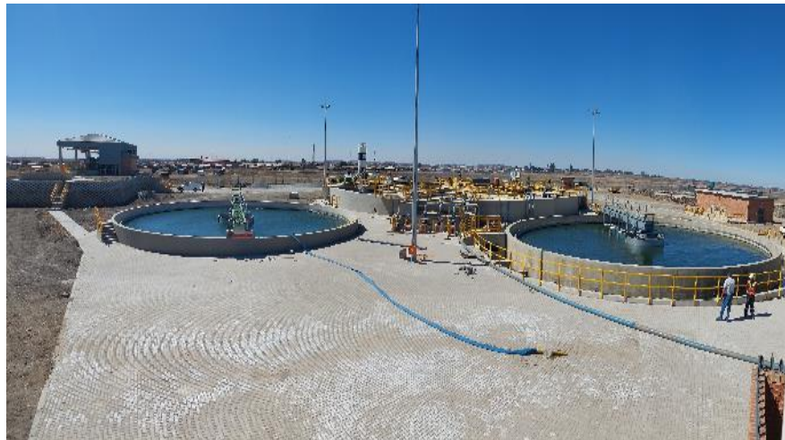
RBIG: Metsimaholo LM - Bulk Sewer Upgrade of Refengkgotso (Deneyville) WWTW Construction complete and Process commissioning is being done
